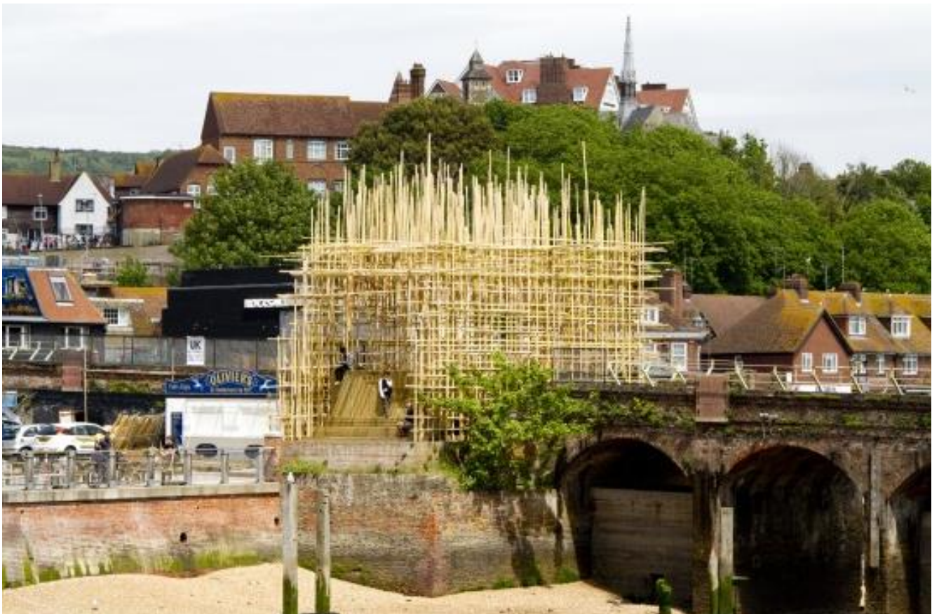
Gabriel Lester The Electrified Line (Cross-track Observation-deck), 2014 Photograph: Gabriel Lester
